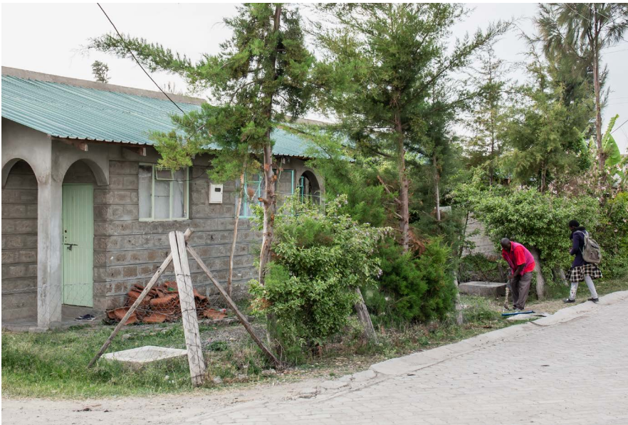
A NACHU affordable housing project site in Nairobi.
